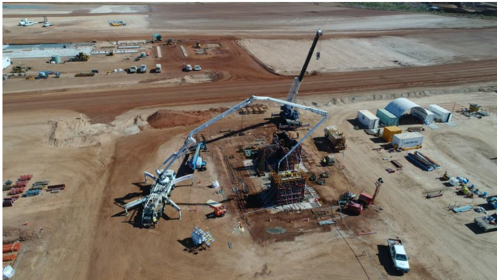
BALL MILL FOOTINGS
