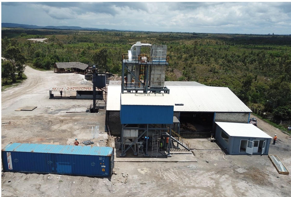
Figure 3: MDS installation completed, electricals in progress.
