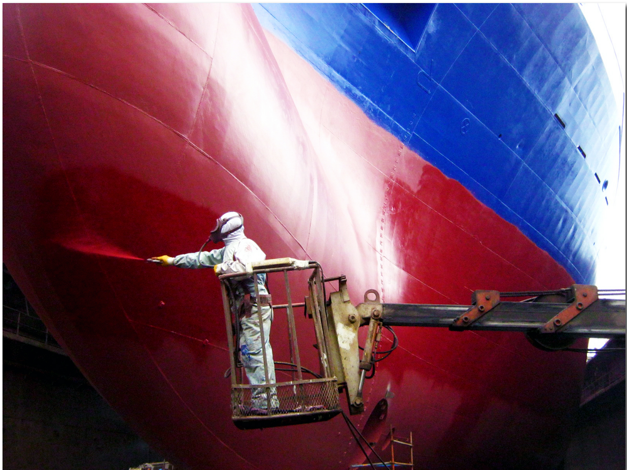
Figure 1 Epoxy based coatings dominate steel protection systems for marine vessels and infrastructure.
