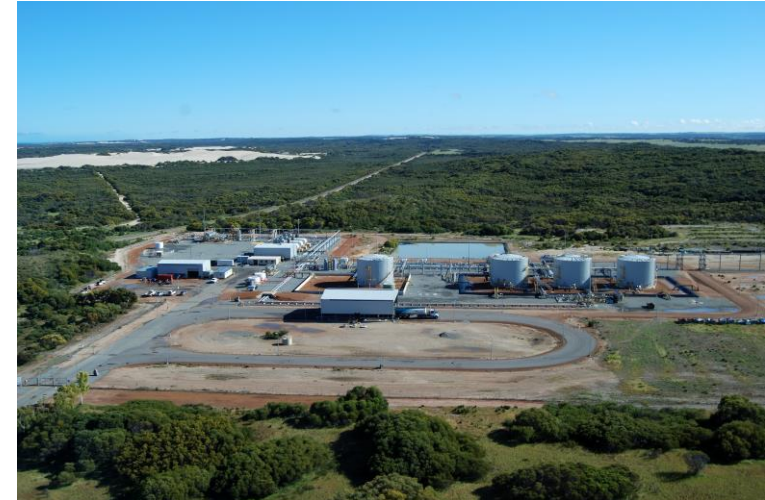
Arrowsmith Stabilisation Plant
