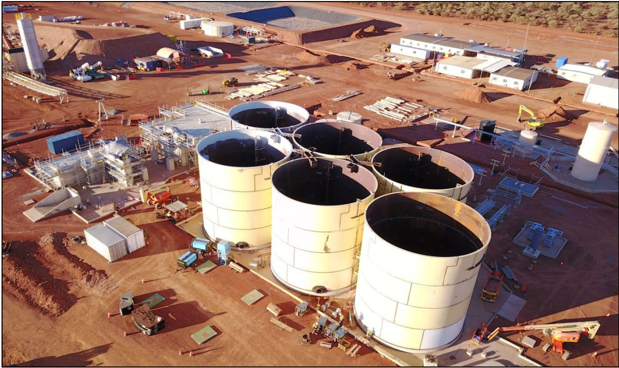
Construction of the Dalgarranga Gold Project Well Advanced
