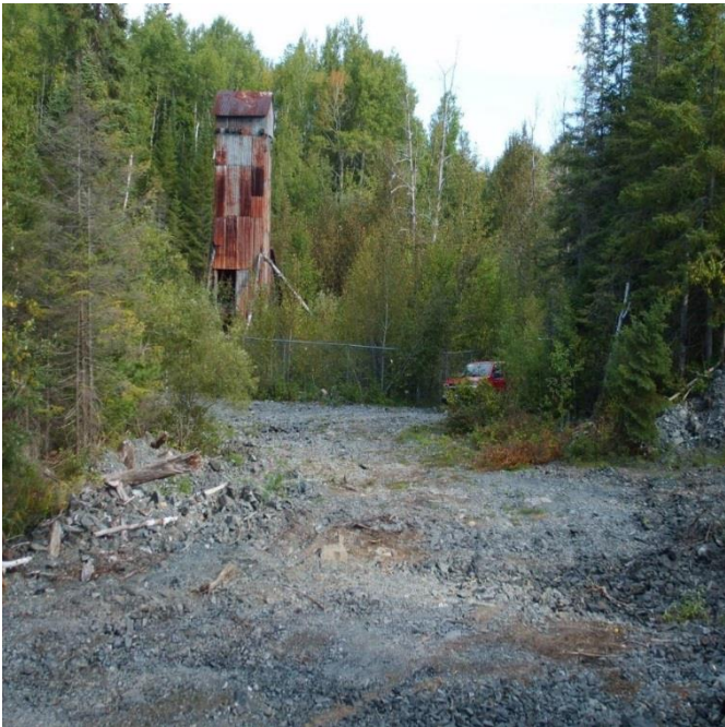
Image 3: Waldman Mine Silver-Cobalt Project – Shaft Entry and historic head-frame
