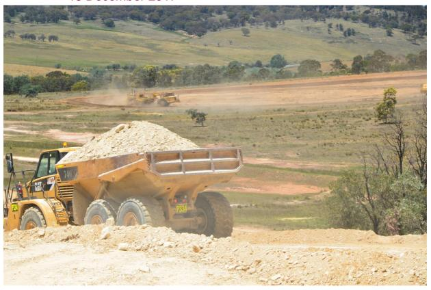
Figure 3: Hauling pad fill in the foreground. Scraper top soil stripping of TSF4 in the background.
