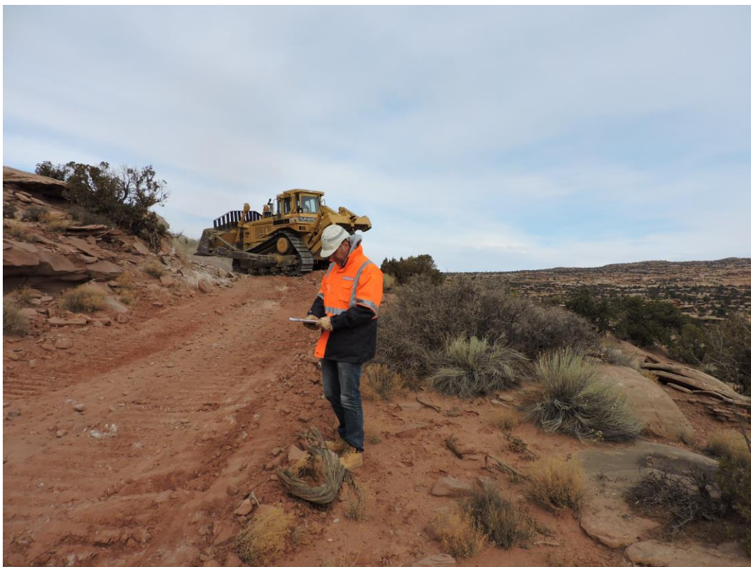
Photo 2: Access Road Upgrade in Progress.
