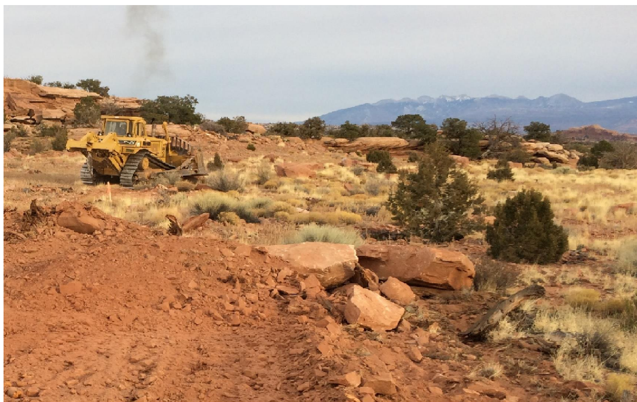
Photo 1: Earthworks in Progress at Anson's Paradox Lithium Project.
