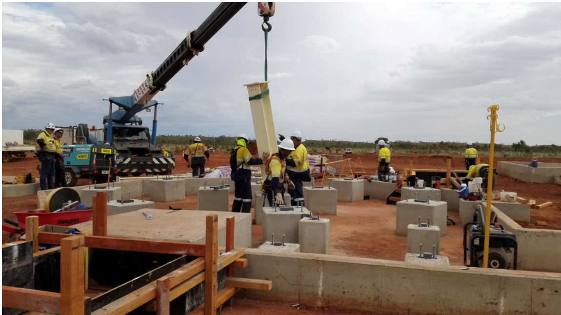
First steel going up at the tailings thickener
