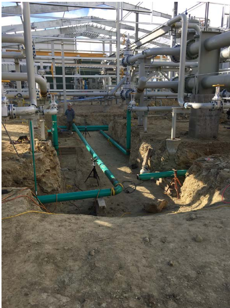
Installing Underground Piping Around Compressor Heat Exchangers – 16 November 2017
