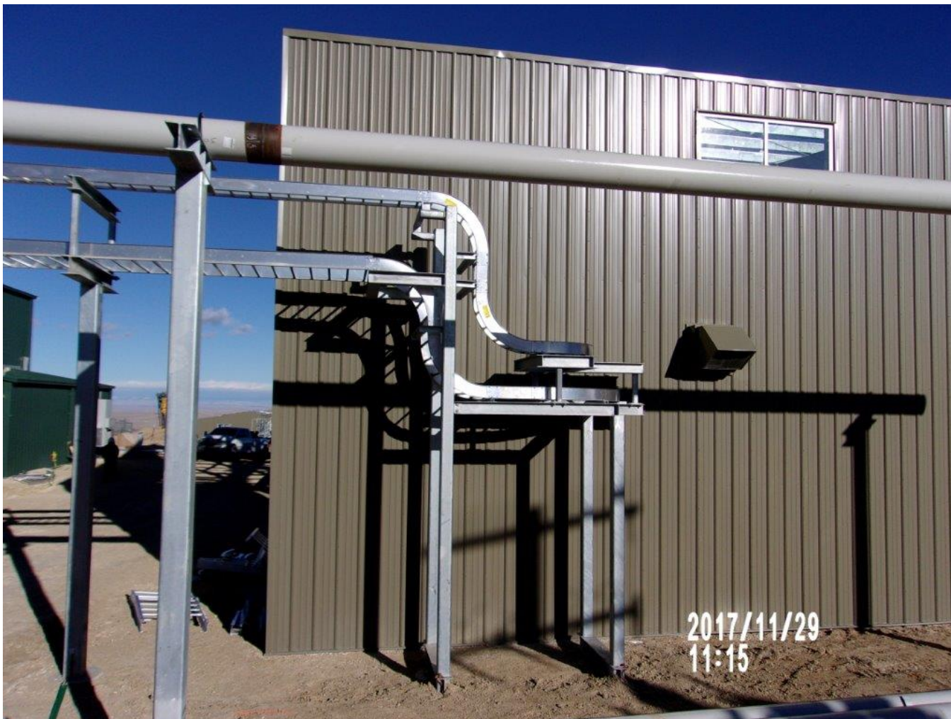
Cable Tray Installation – 30 November 2017
