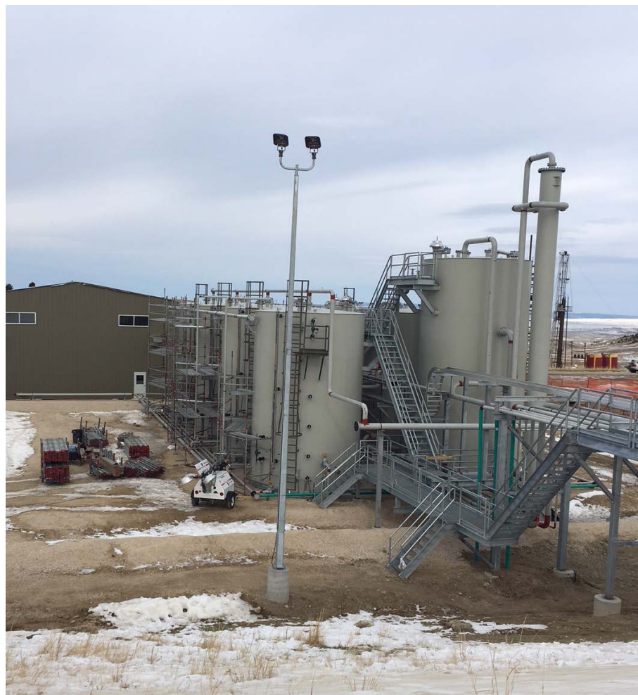
Tank Farm and Pump Area – Scaffolding for Insulators –14 December 2017
