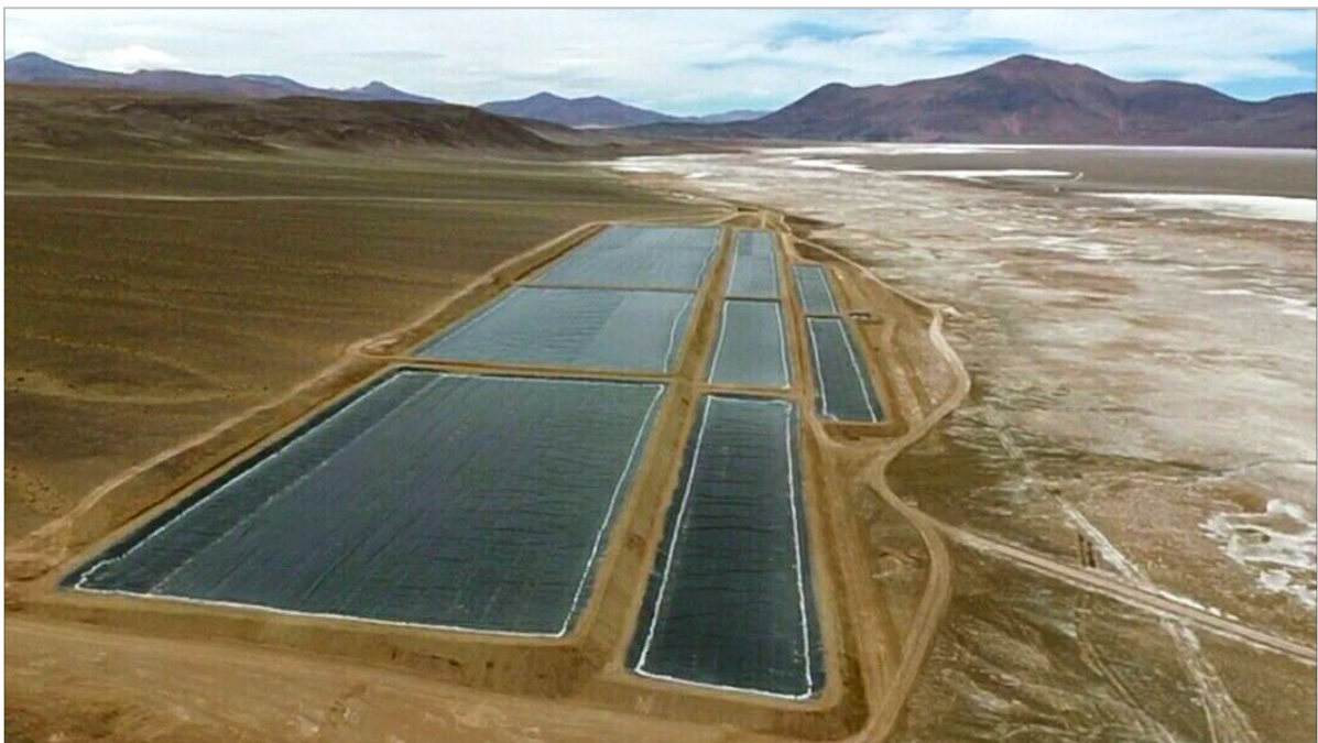
Photos 2 - 3. Rincon Lithium Project – initial Stage 2 Evaporation Ponds
