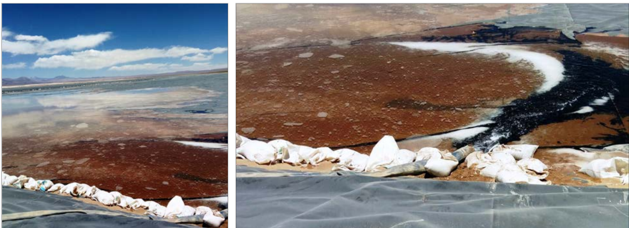
Photos 1 - 2. Rincon Lithium Project – Brine Pumping into Stage 2 Evaporation Ponds
