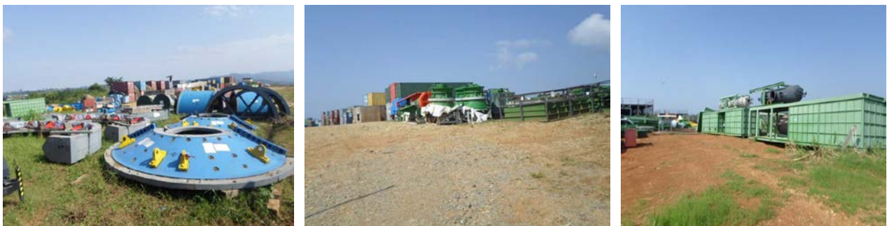
Figure 7, 8 and 9: Mechanical plant and equipment at the Project site contained within 115 sea containers
