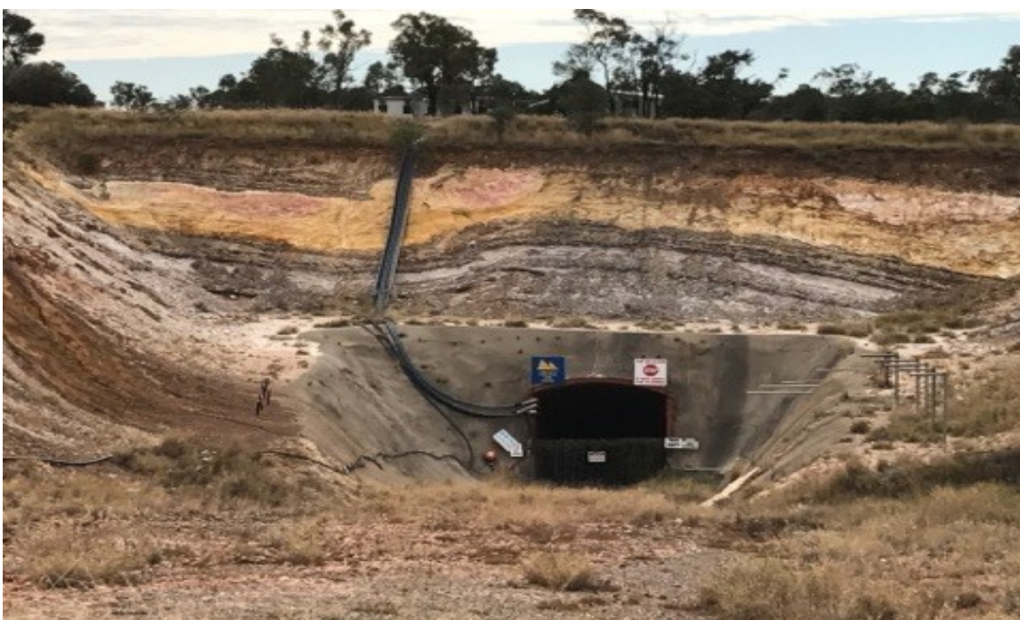
Figure 5: Portal to underground workings. Historical production was 72,979 t @10.01g/t for 23,490 ounces.
