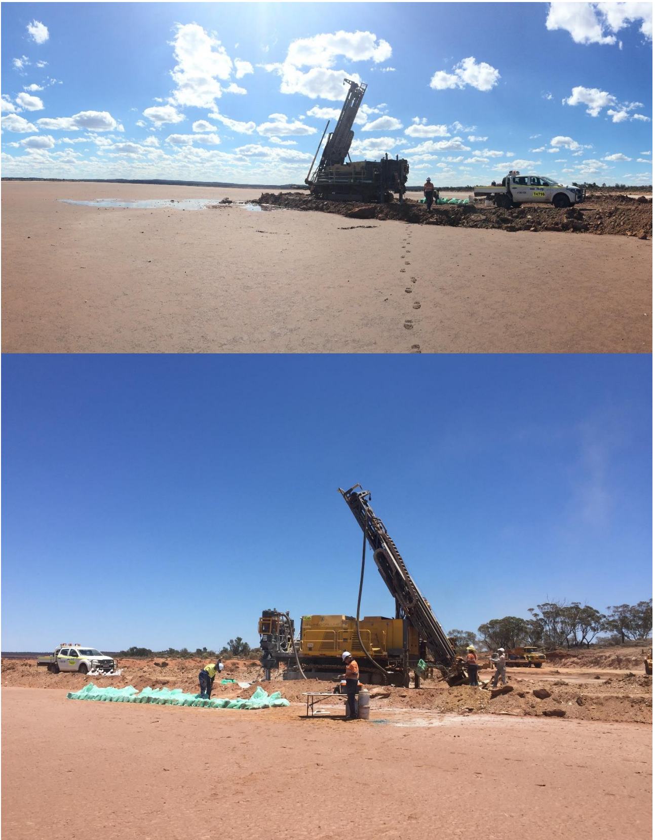
Figure 2. Drilling at Slate Dam, December 2017.
