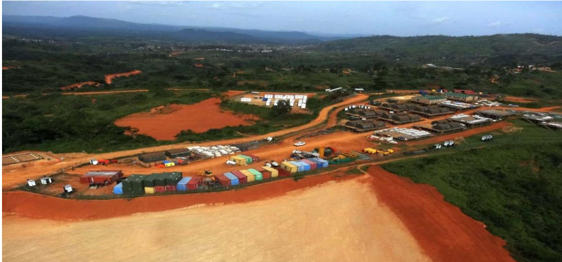
Figure 1: The Adidi-Kanga Gold Mine - Mongbwalu Gold Project Development Site located on Mining License PE5105
