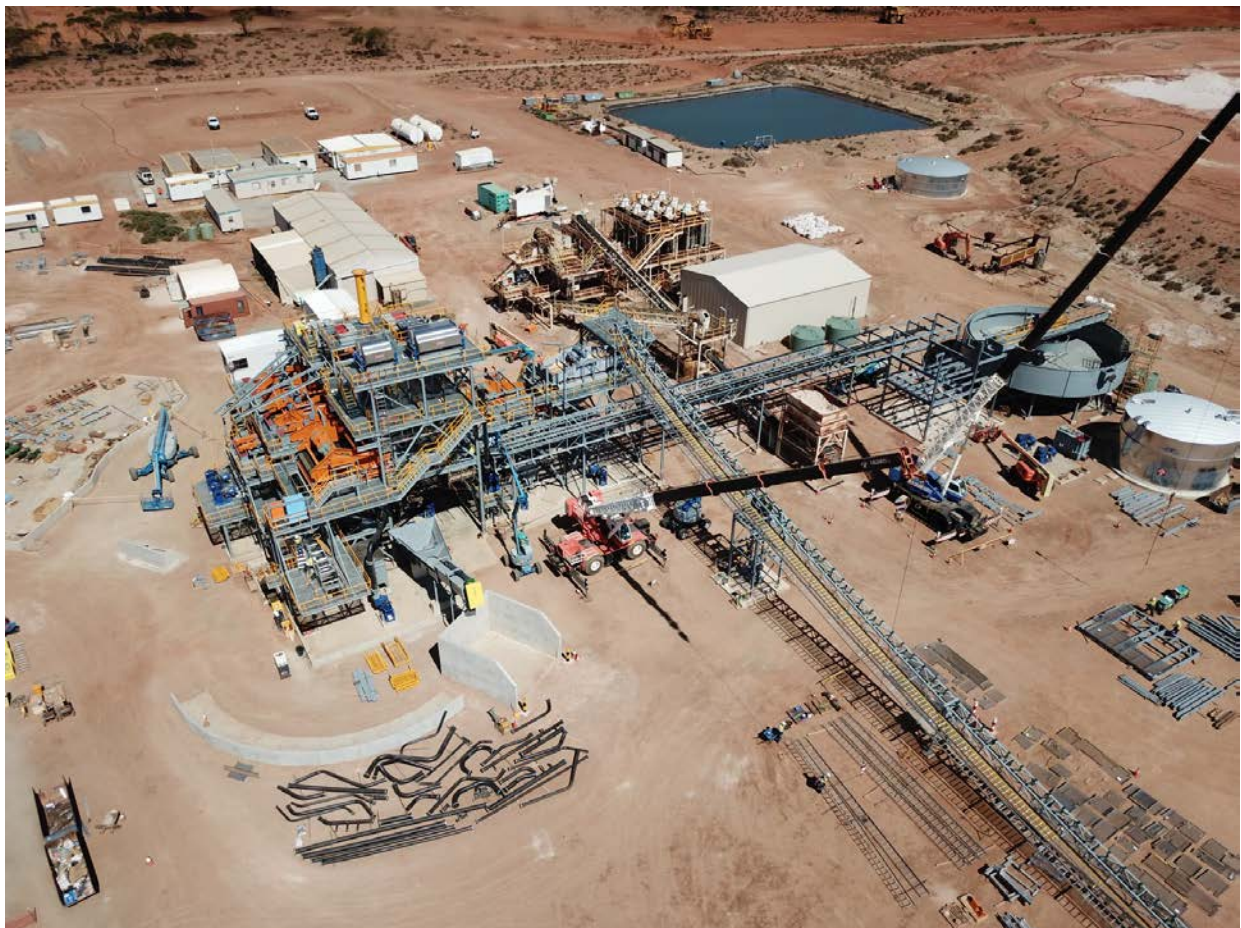
Figure 2 | Plant overview (DMS in foreground) - December 2017
