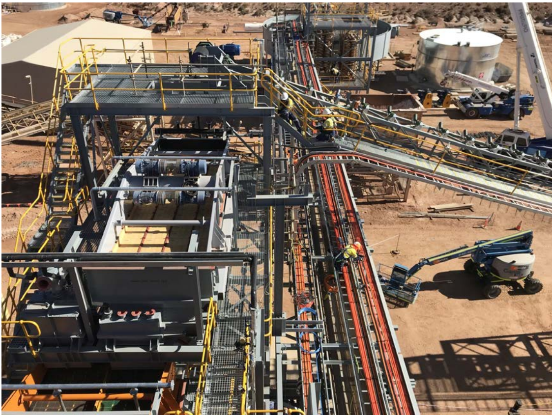
Figure 4 | Piping and Electrical Work – January 2018
