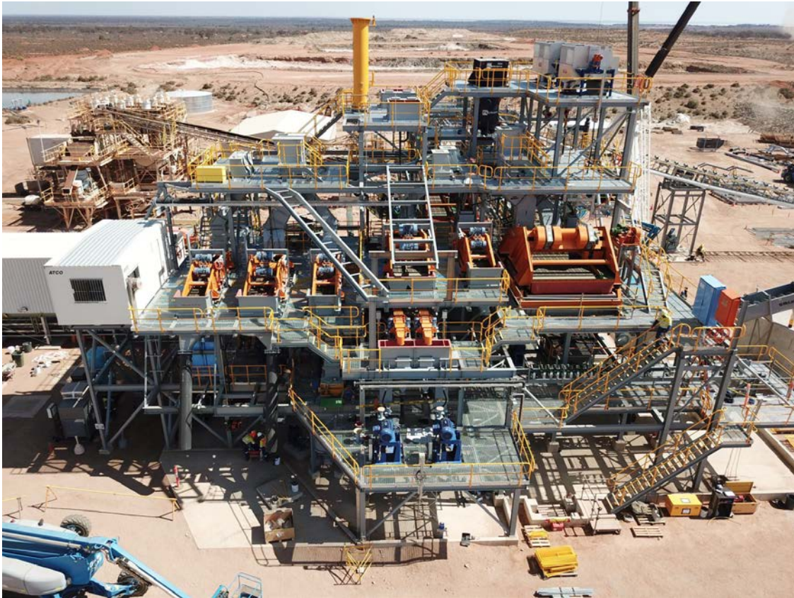
Figure 3 | DMS Plant – December 2017
