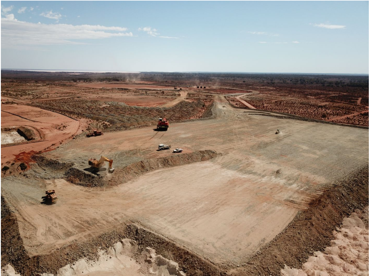
Figure 7 | ROM and crusher pad – December 2017
