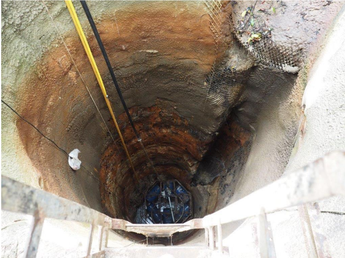
Image 5; Cuca shaft de watering as at 10 January 2018
