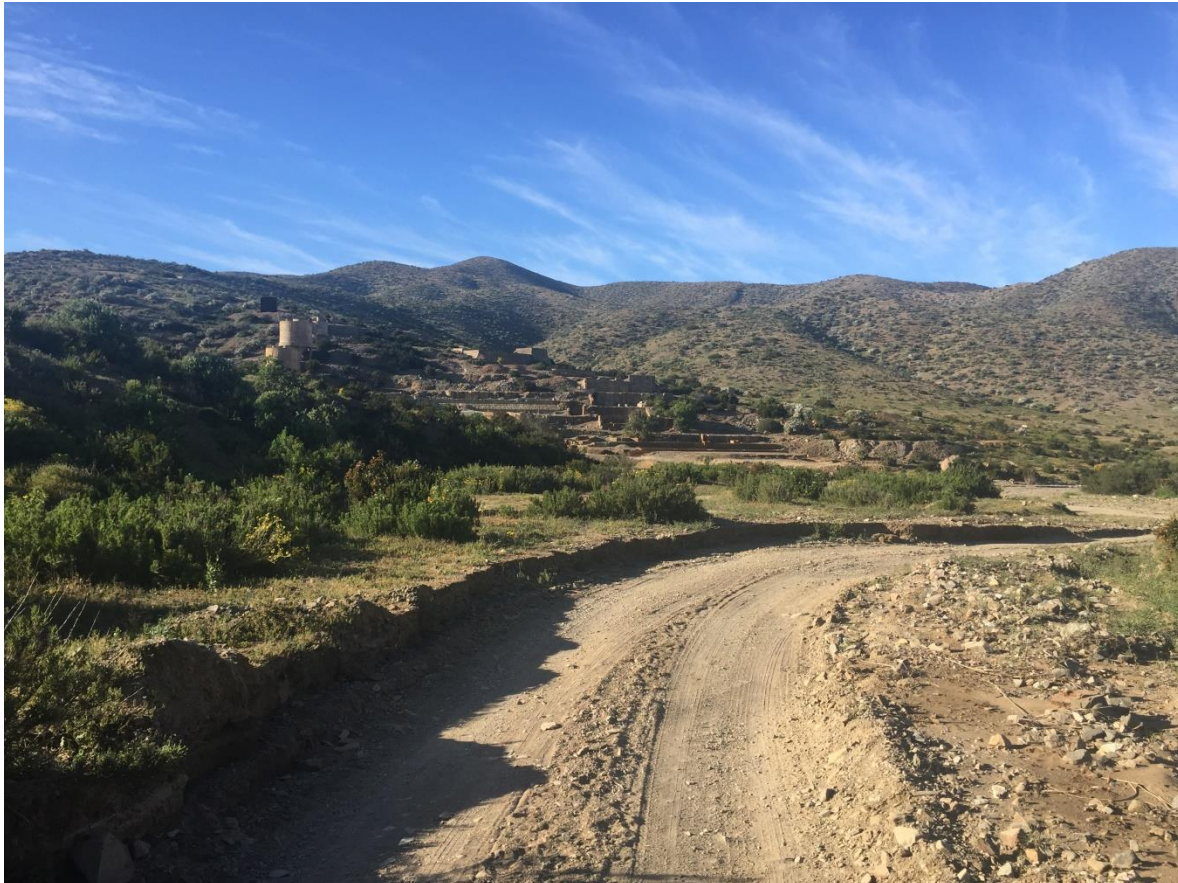
Figure 2. Historic La Cobaltera Processing Plant (processed cobalt ores only)
