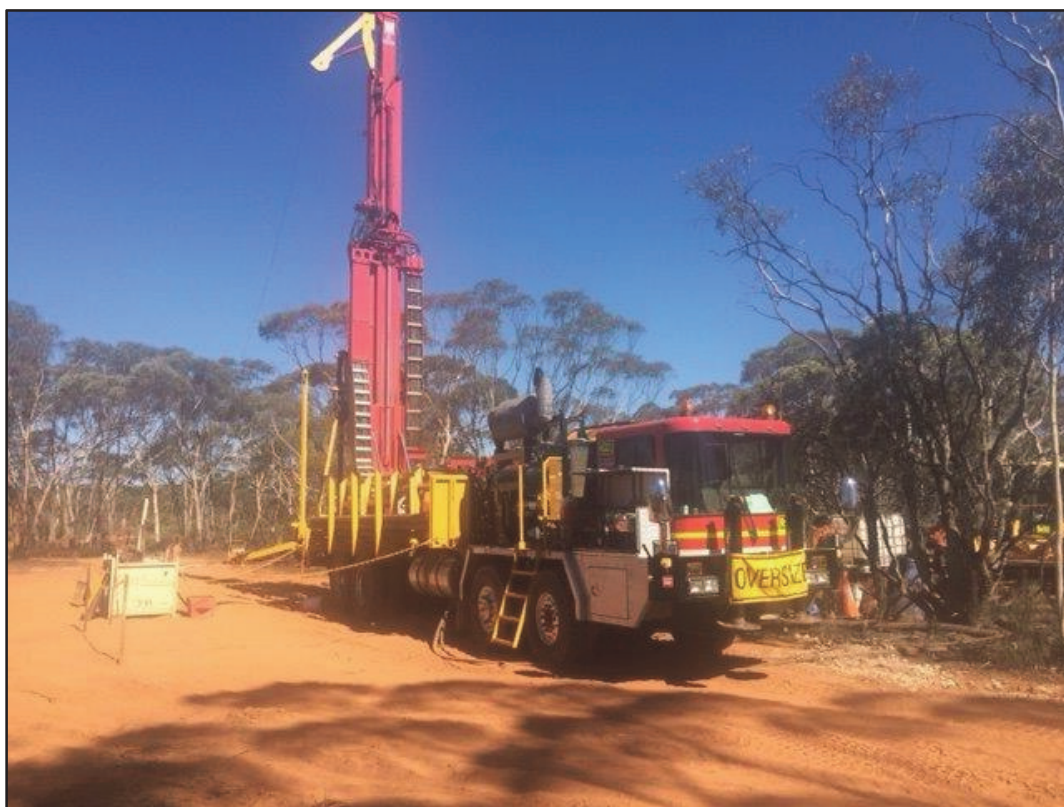
Figure 5: Aquadrill Water Bore Rig – 12 January 2018
