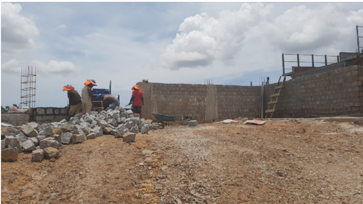
Feeding ramp safety-wall started.
