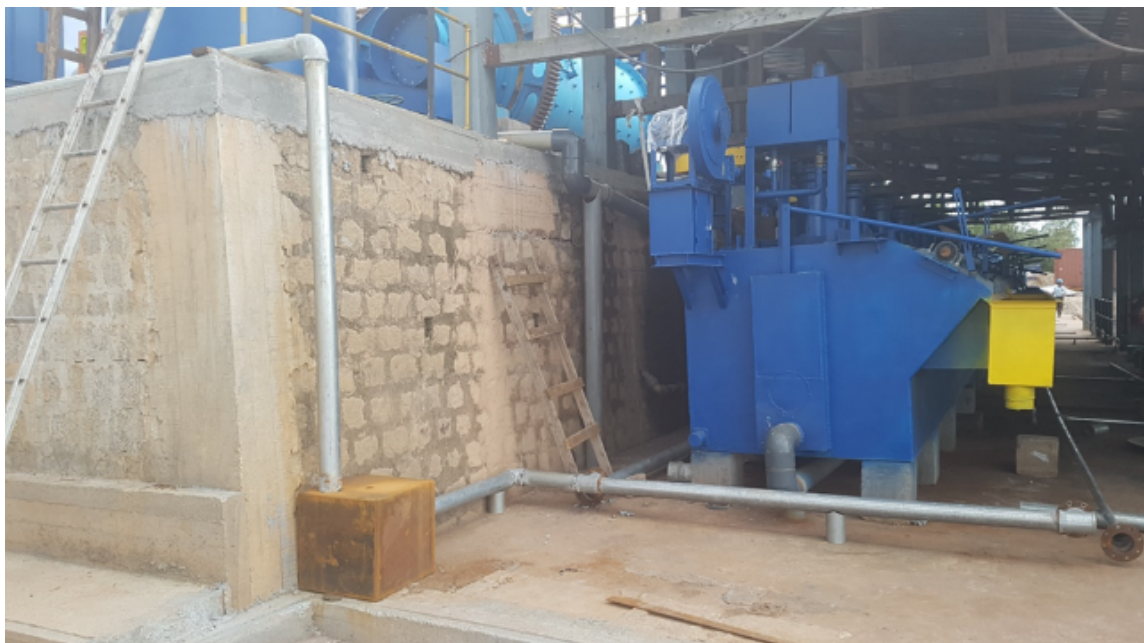
Water piping and manifold installation nears completion.
