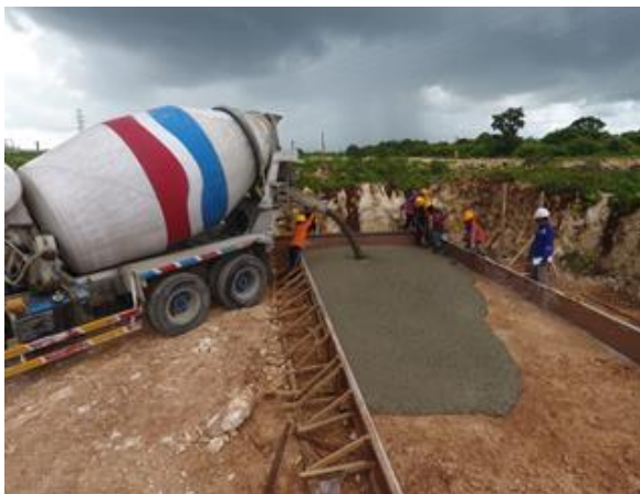
Concrete levelling slabs being poured
