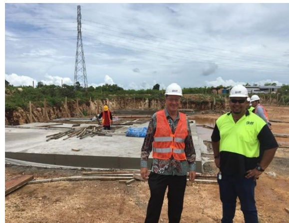
Hamish Bohannan (MD & CEO) and John Pilotti (Electrical Projects Engineer) at the Kupang Smelting Hub Site.
