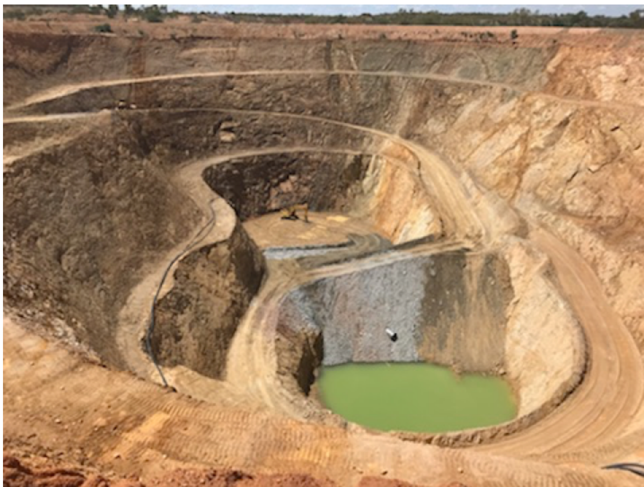
Wagtail North pit with the portal platform, in-pit sump and new access ramp established for underground development.
