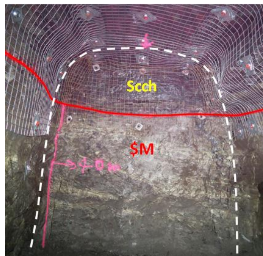
774 ore drive (4.0mW x 3.5mH) with a face grade of 9.7% nickel
