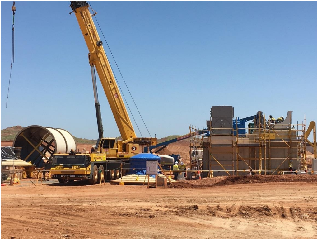
Figure 4 – Ball Mill assembly
