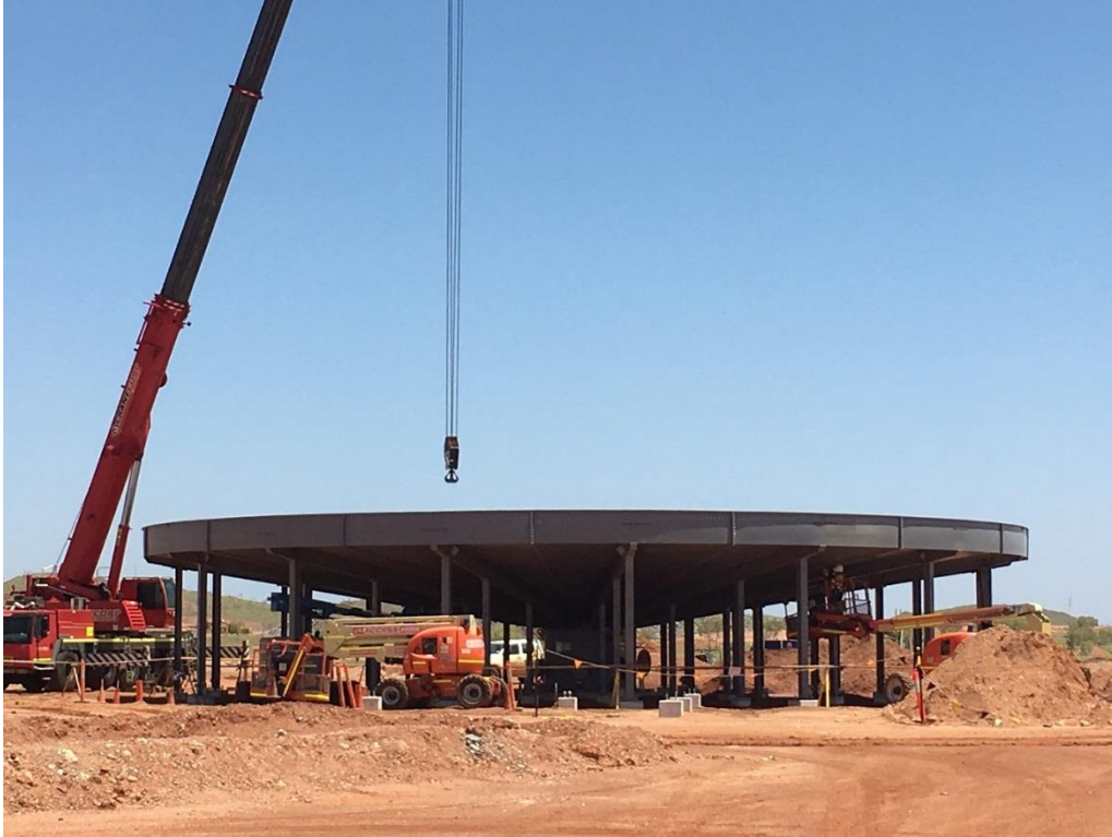
Figure 3 – Tailings thickener steel erection
