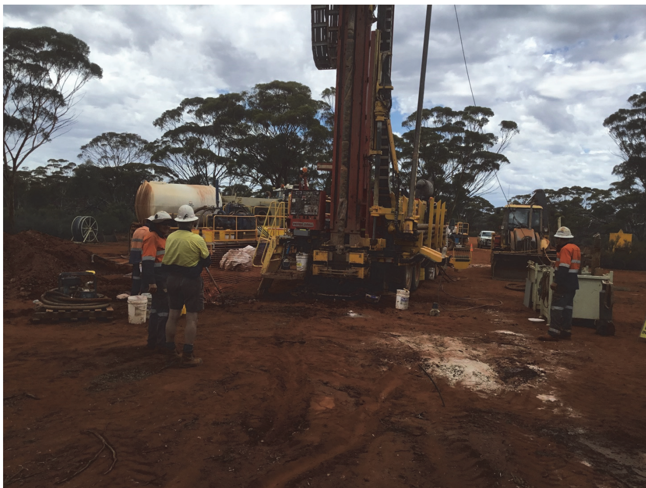
Figure 5: Project Manager Alex McCulloch conferring with Drill Foreman Scott Baily at production water bore 2 kms east of lost dog ore resource
