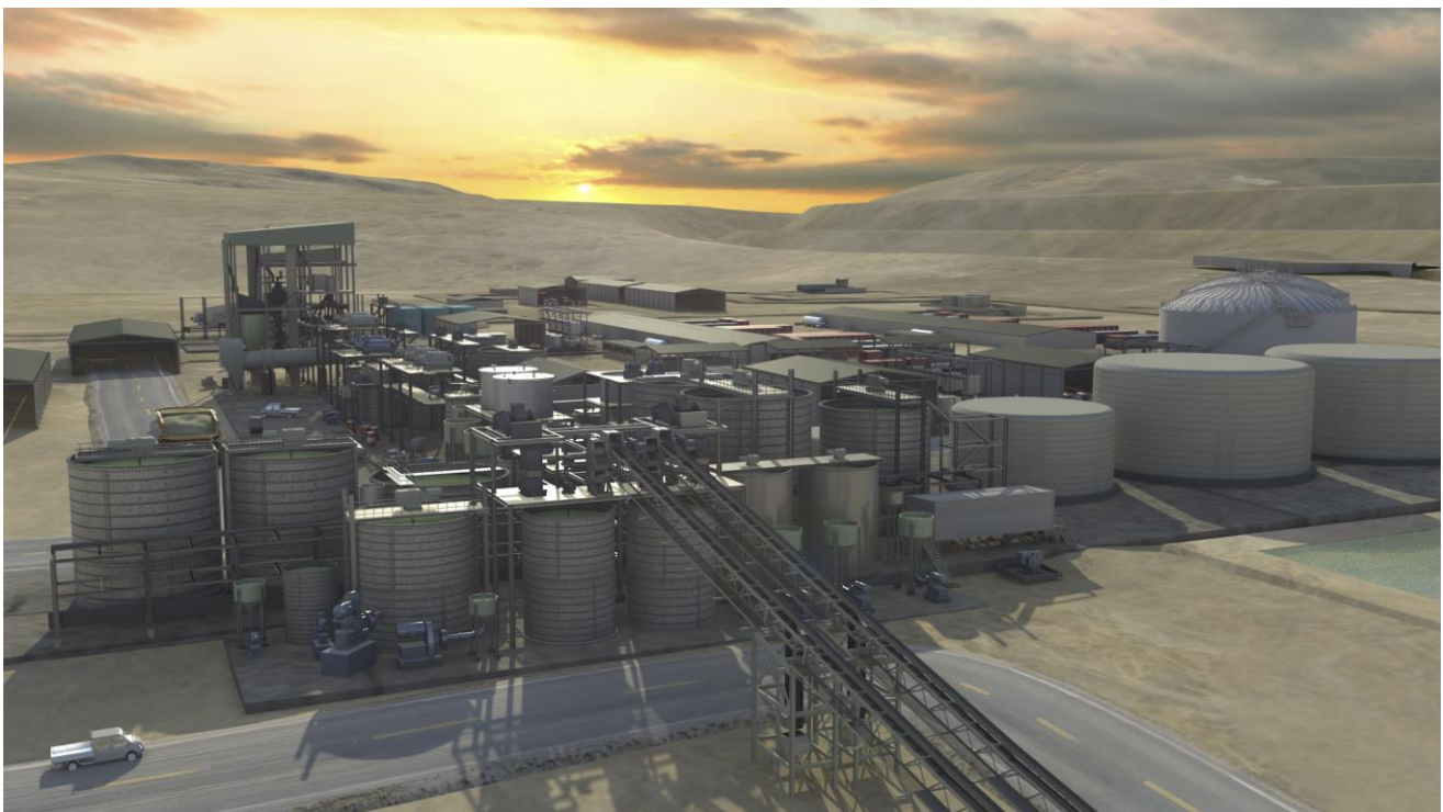
Figure 5: Colluli processing plant viewed from the run-of-mine pad
