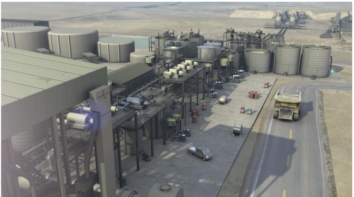
Figure 1: Colluli processing plant looking out to the run-of-mine pad
