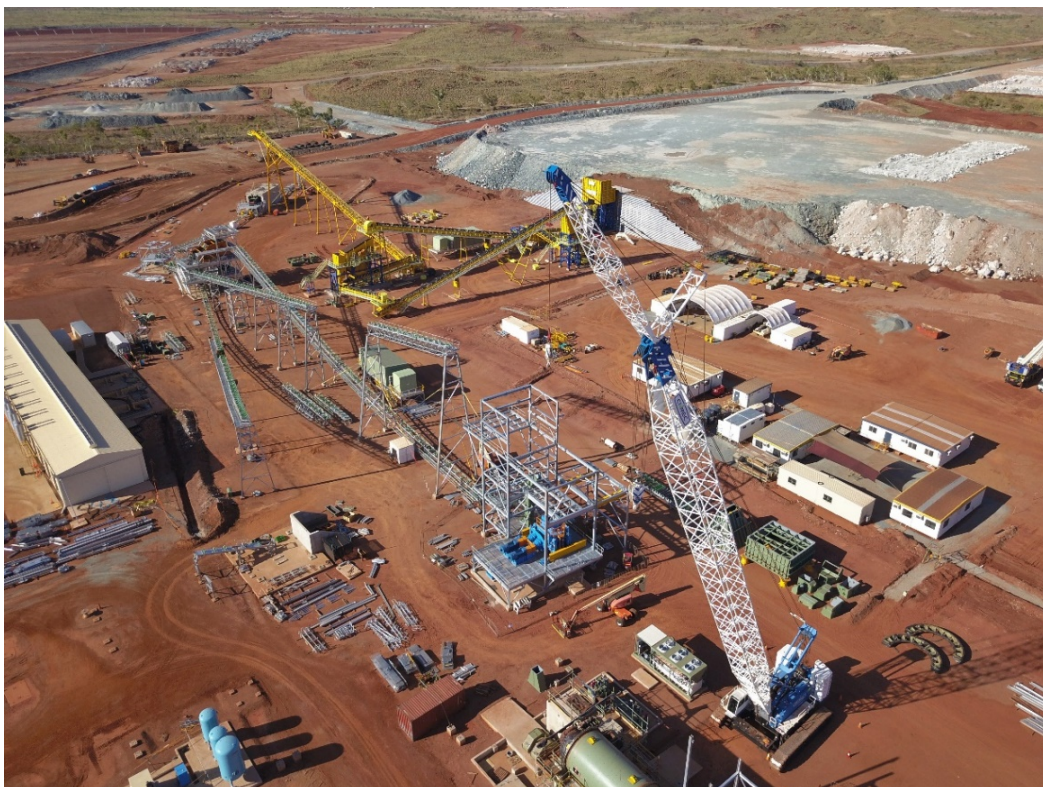
Mine site works nearing completion on the Altura Lithium Project
