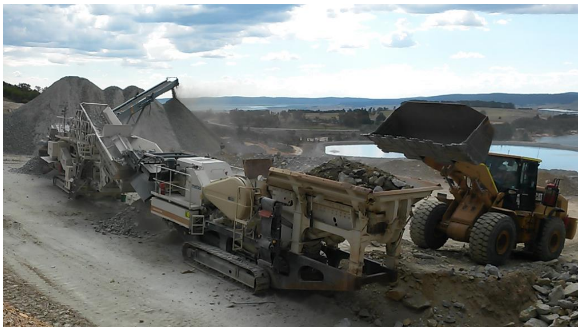
Figure 3: Crushing of material for final pad pavement
