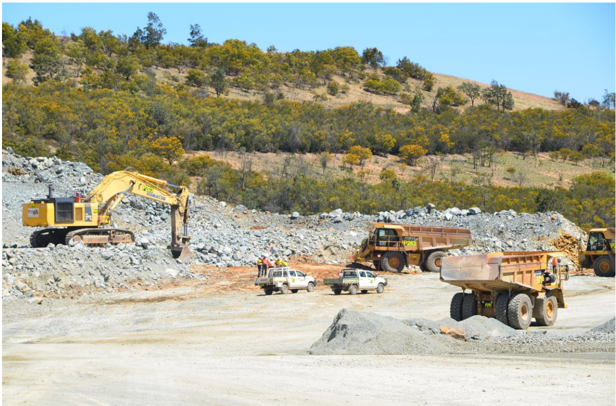
Figure 5: Clearing of underground box cut area
