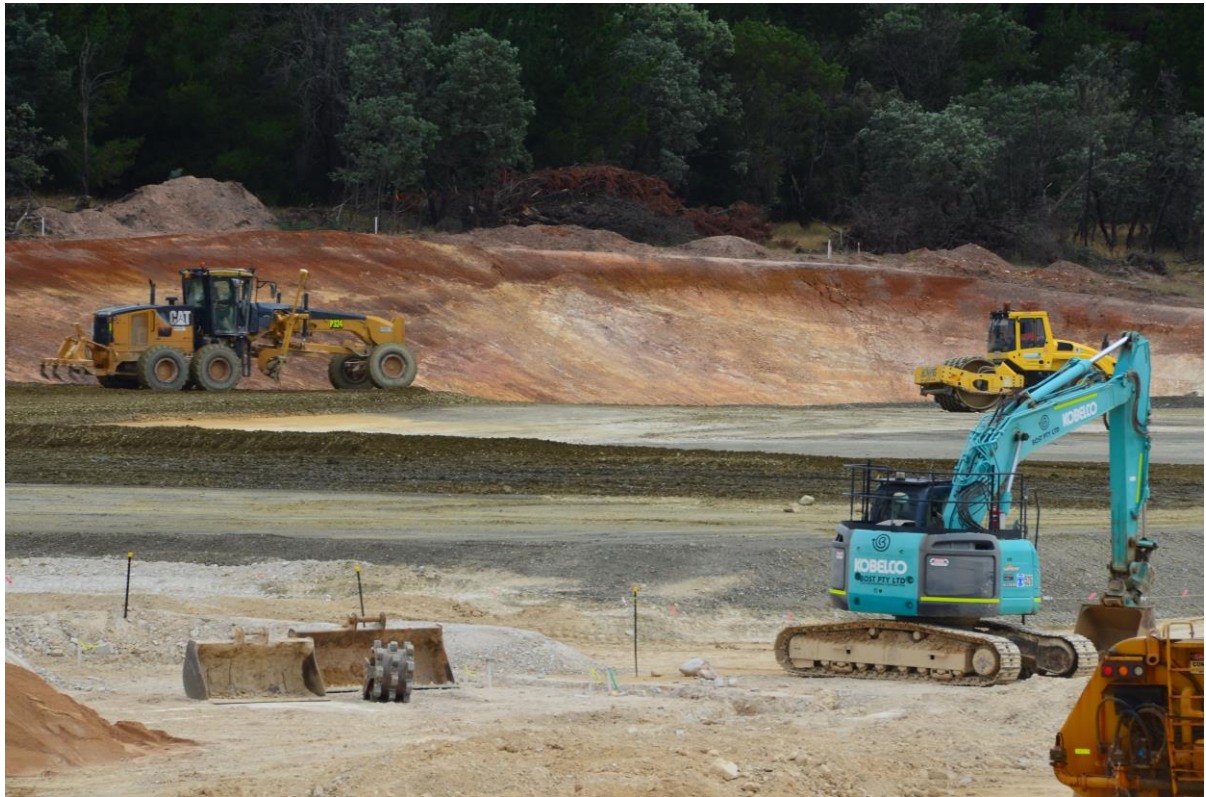
Figure 4: Final pavement being placed on process plant pad
