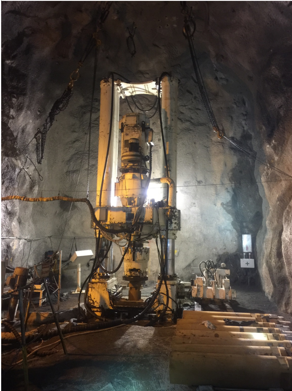
Figure 1: Ventilation raisebore drilling at the Syama Underground mine
