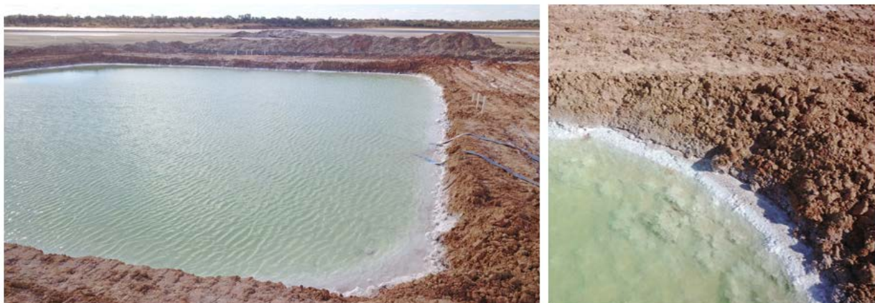
Figure 5: Pond 3 with Salt Deposits Forming
