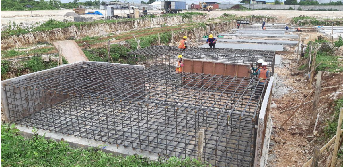
Figure 1: Concrete foundations for the Smelting Hub at Bolok Industrial Estate
