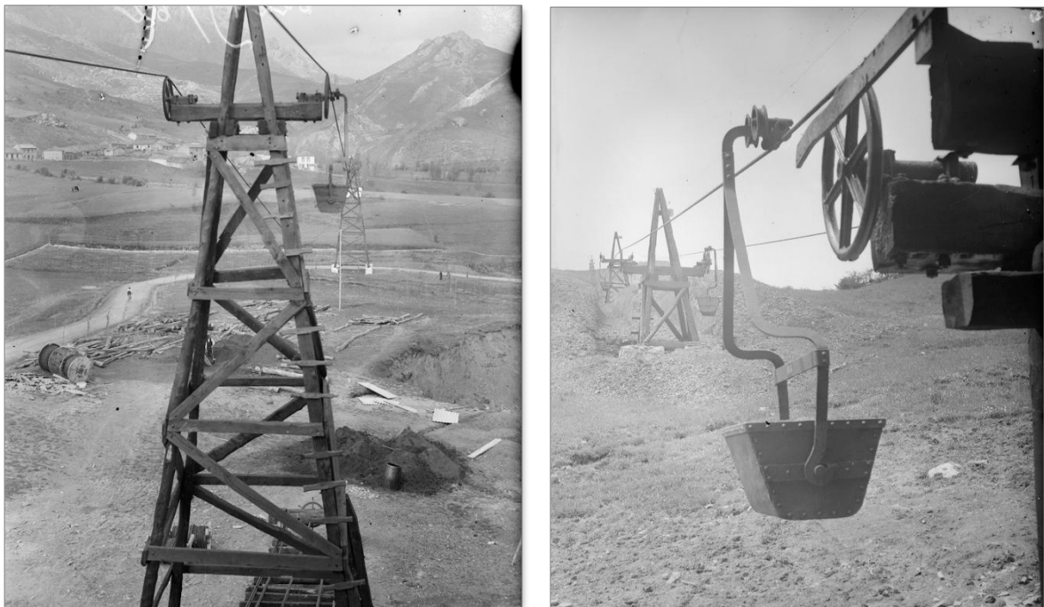
Figures 3 & 4 – Aerial ropeway & ore delivery buckets from La Profunda to Villamanín plant (circa 1920s)
