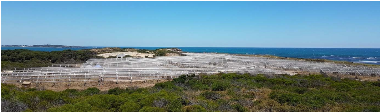
Garden Island Microgrid 2MW solar farm construction – solar frames complete
