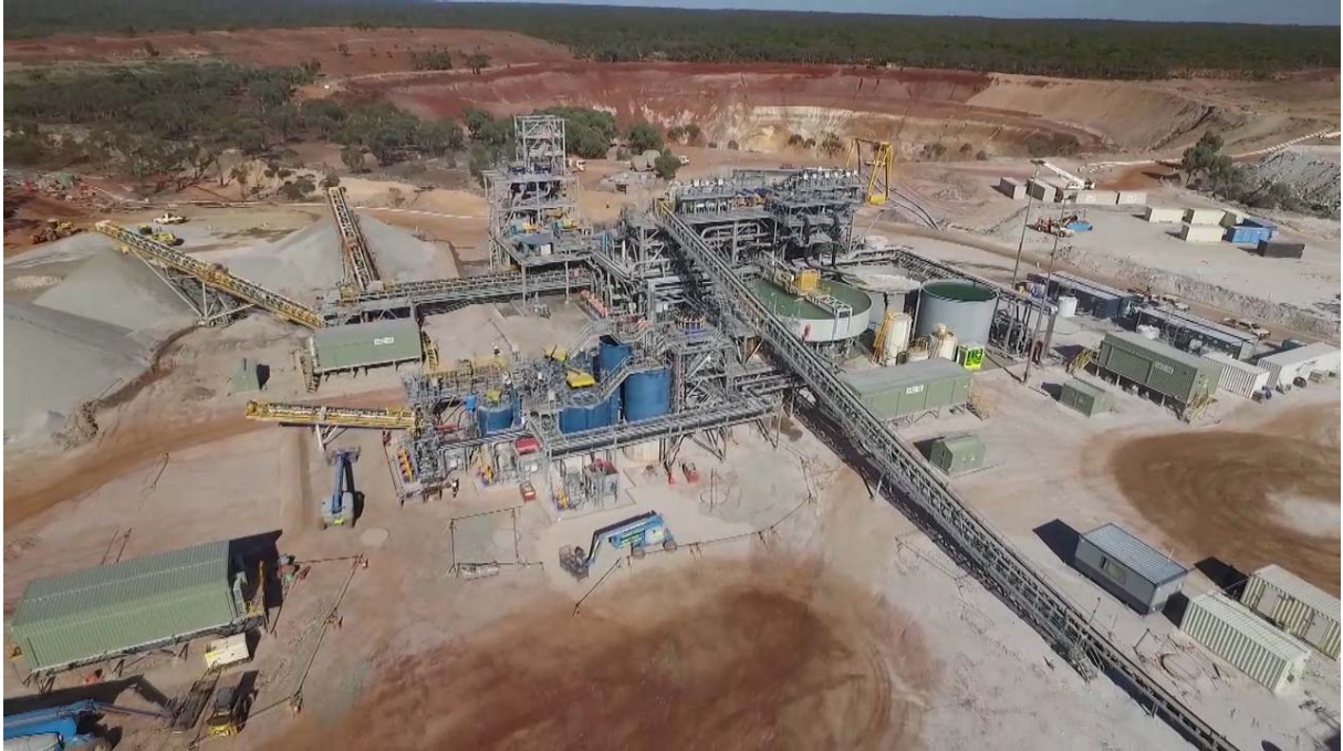
Image 1: Aerial View of Mt Marion Lithium Operation's Processing and Tailings Storage Facilities
