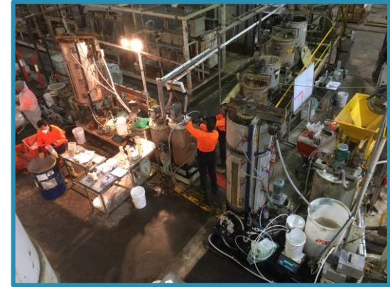
Bulk Pre-Leach Pilot Plant
