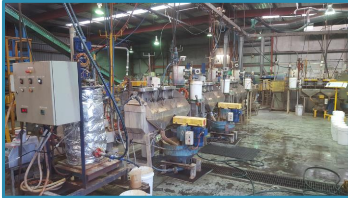
Beneficiation Pilot Plant
