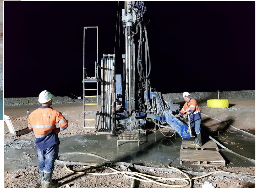
Grouting rig in action, night shift February 2018
