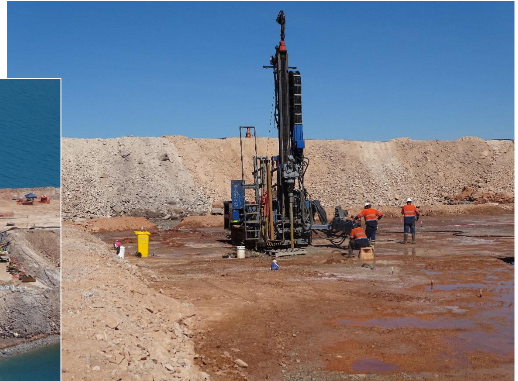
Drilling vertical drains, August 2017
