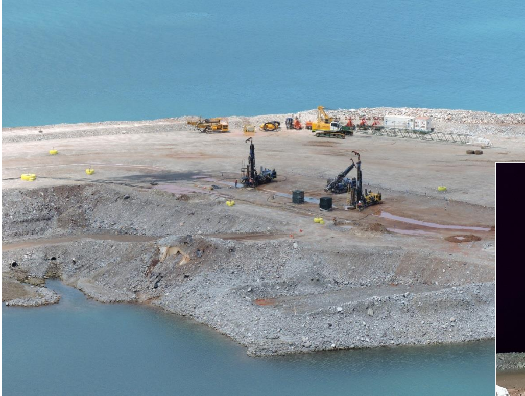
Grouting rigs working at western end of embankment, January 2018
