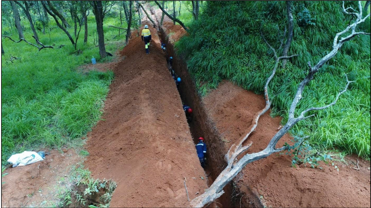
Figure 3: Trenches being excavated at Monwezi 2 ahead of diamond drilling
