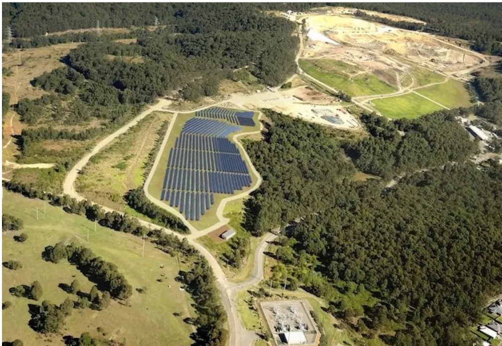
Impression of the completed Solar Farm
