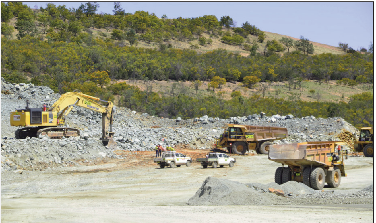
Figure 5: Clearing of underground box cut area
