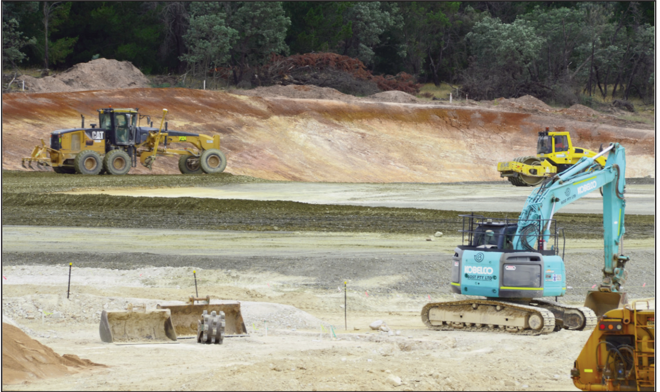
Figure 4: Final pavement being placed on process plant pad
