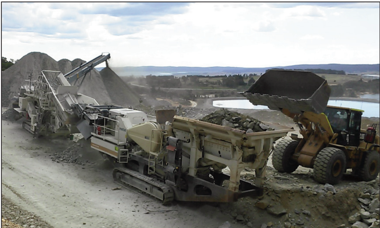
Figure 3: Crushing of material for final pad pavement
