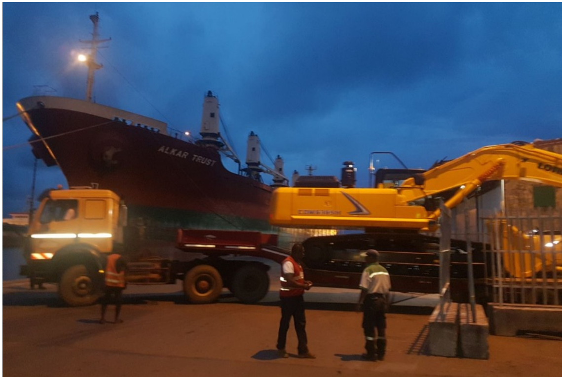
New Excavator delivered, commissioned and put to work.
