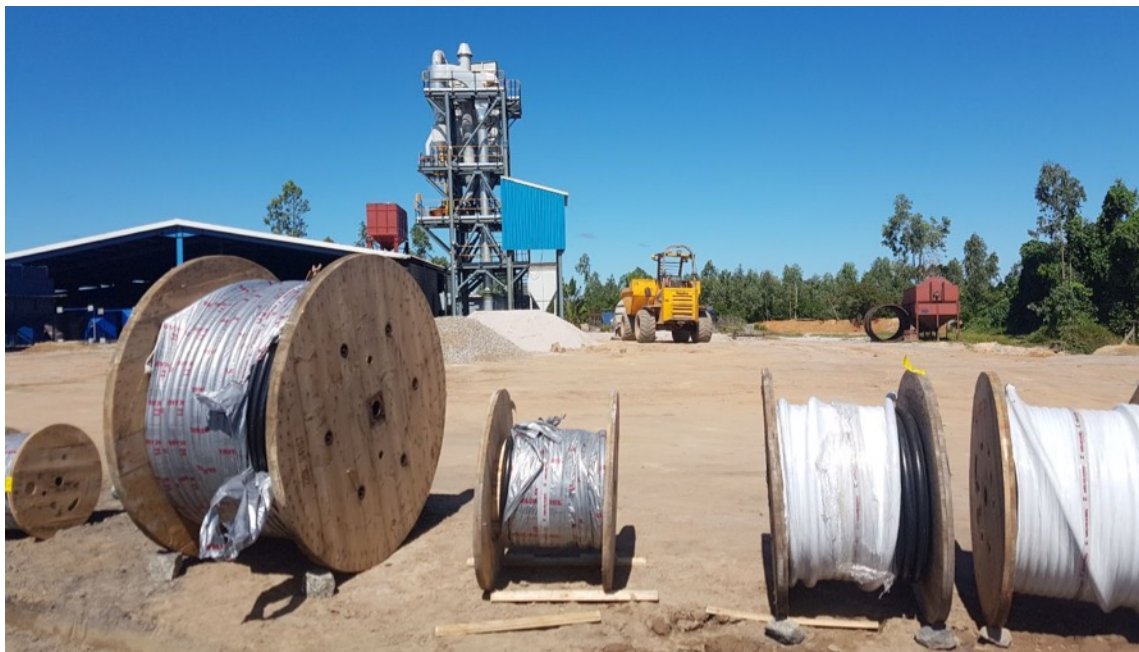
Delivery of electrical components for the completion of Stage 1.
