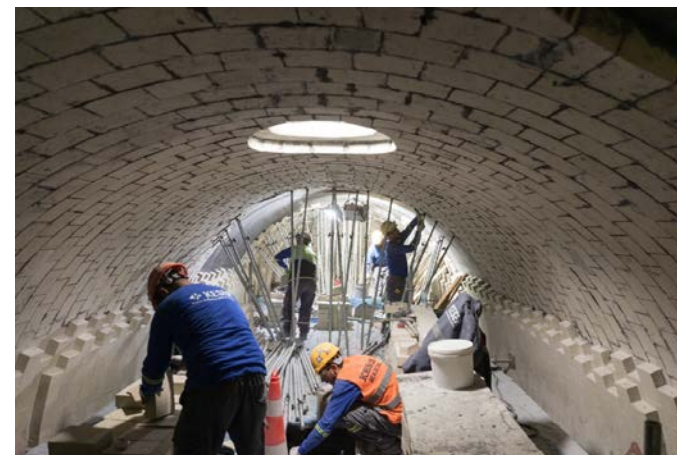
Autoclave Brick Lining
