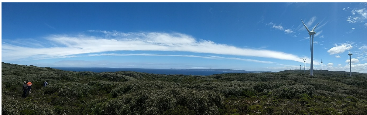
Onshore Site Inspections and Surveys in Albany
