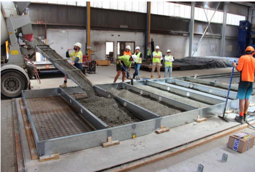
Images showing casting of lightweight slab panels to assess the manufacturing process.
