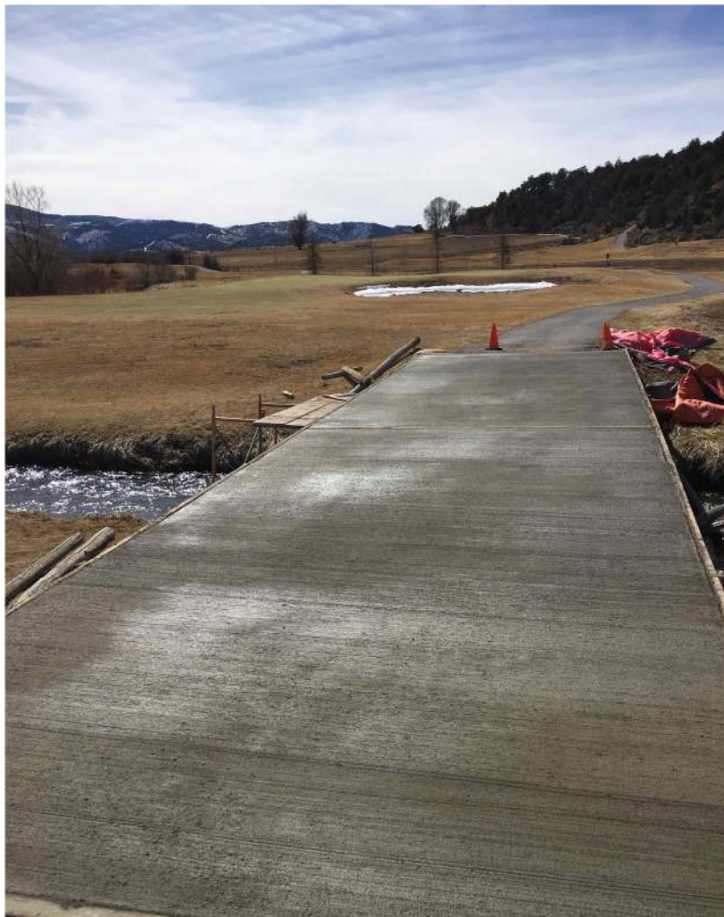
Figure 5. Gypsum Golf Course Bridge Project
