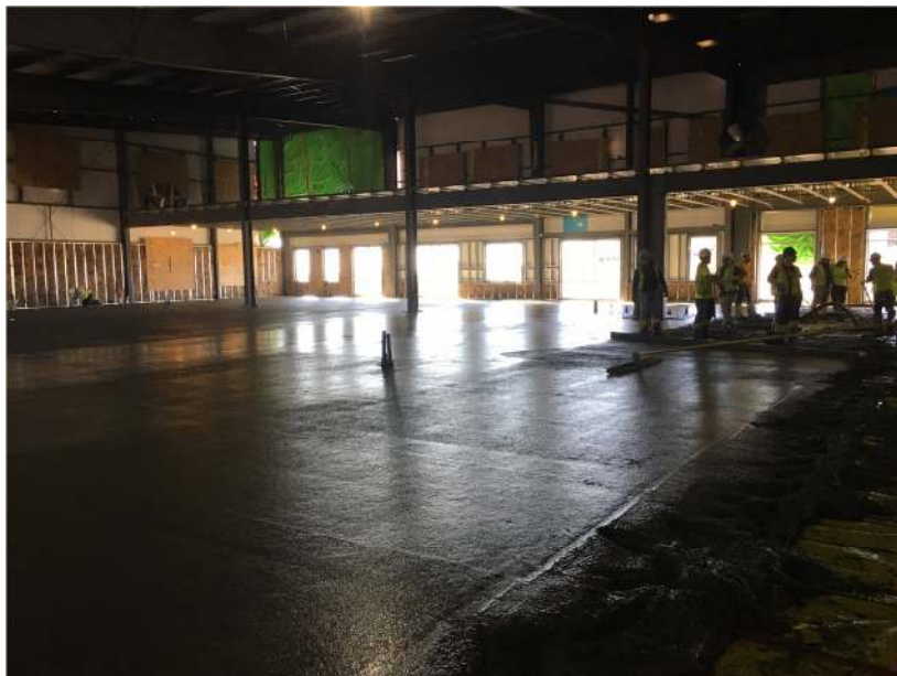
Figure 2. New factory concrete floor being poured
