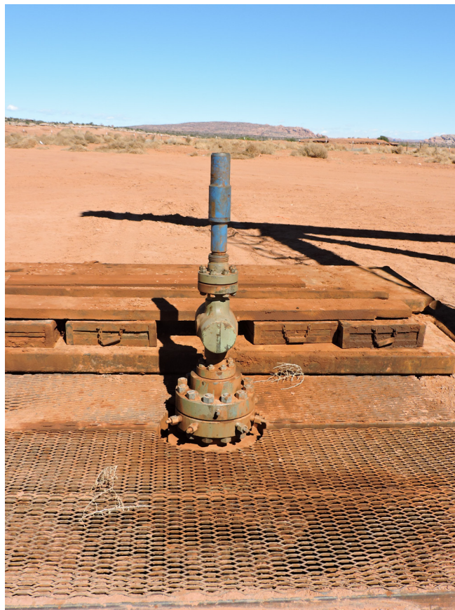
Figure 1: The Cane Creek well ready for the work over sampling program.
