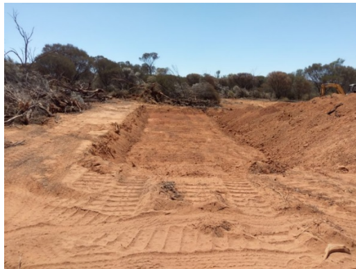
Figure 10. Excavation at Mertondale for some of the large nuggets including the 21oz nugget
