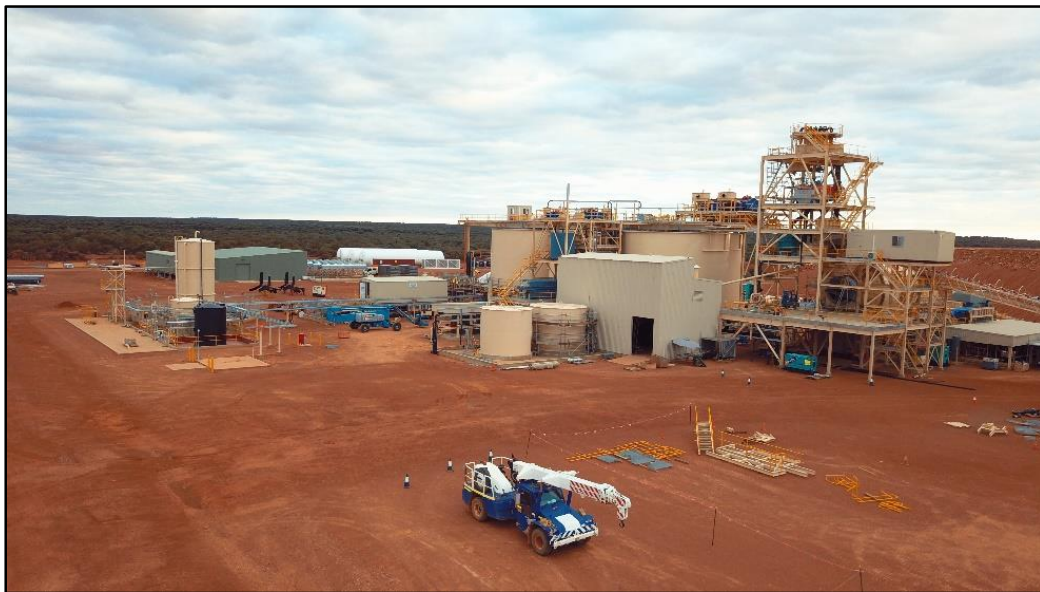
Photo 4: Cyclone Tower Construction Complete and Installation of Mechanical equipment - Well Advanced
