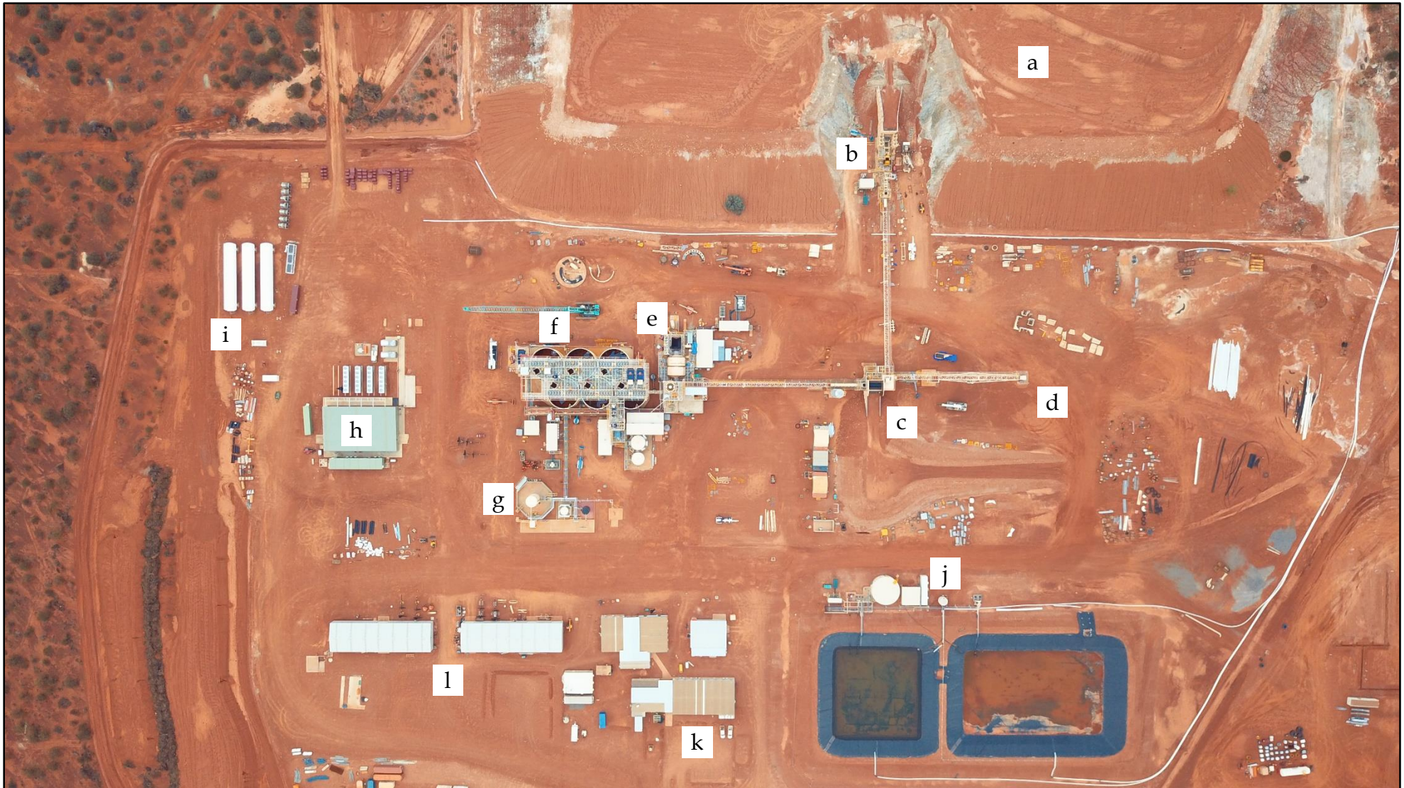
Photo 2: Dalgara Process Plant Site Overview
