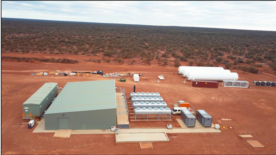
Photo 6: Zenith's Engine Hall and HV Switchroom & EVOL's LNG Storage Facility
