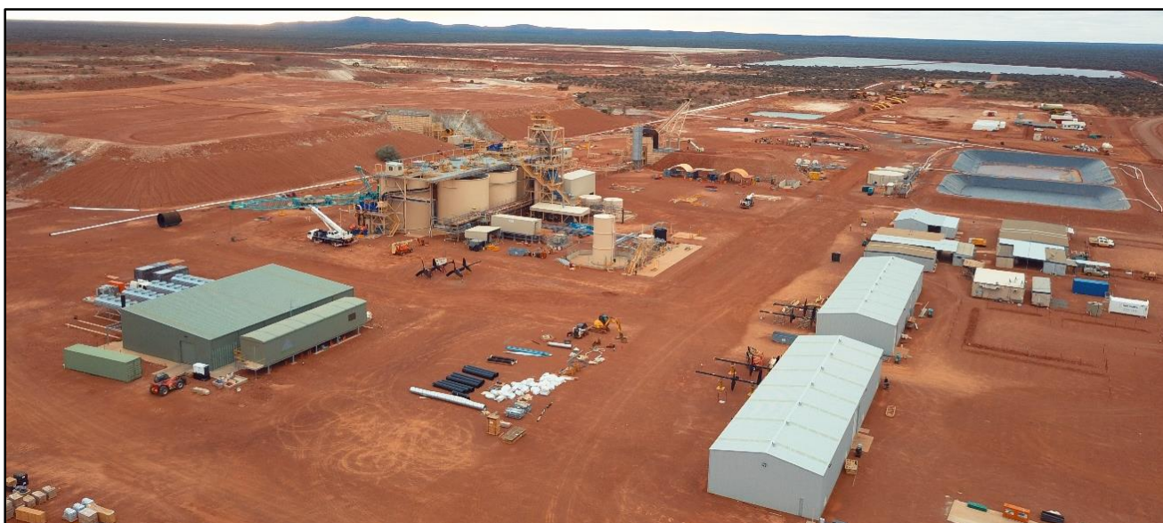
Photo 1: Dalgarranga Plant Site Construction Progress
