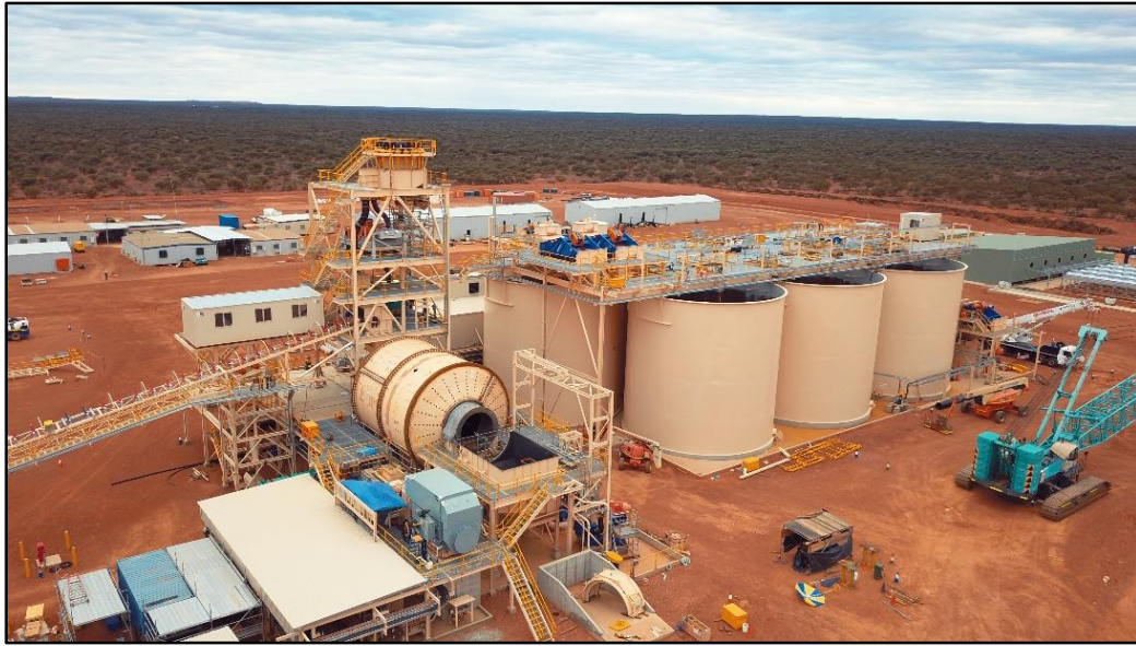
Photo 3: SAG Mill Installation – Progressing Well
