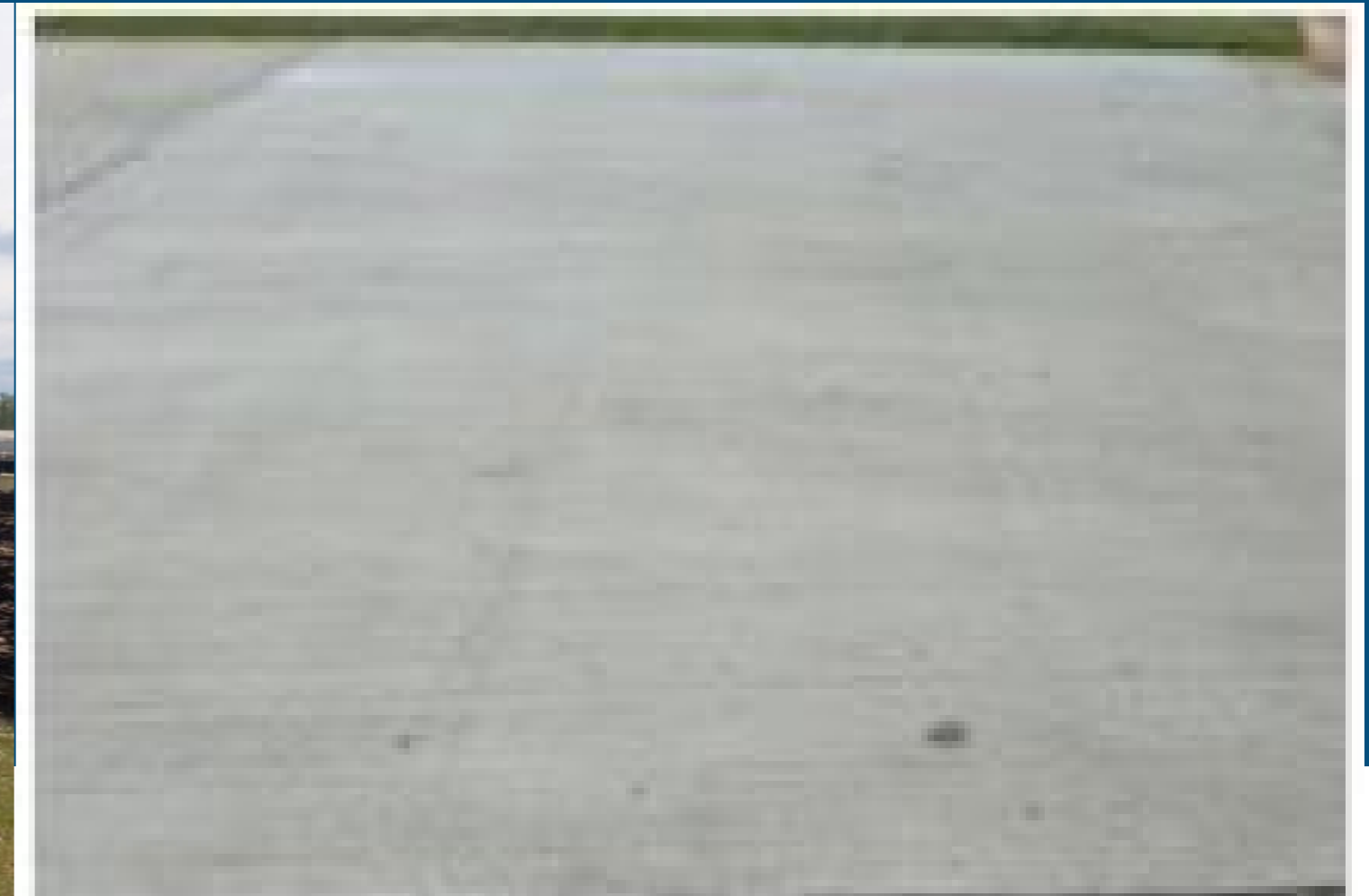
EdenCrete® TRIAL SLAB
