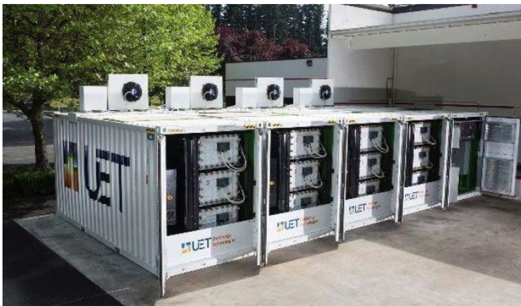
Vanadium redox flow battery storage
