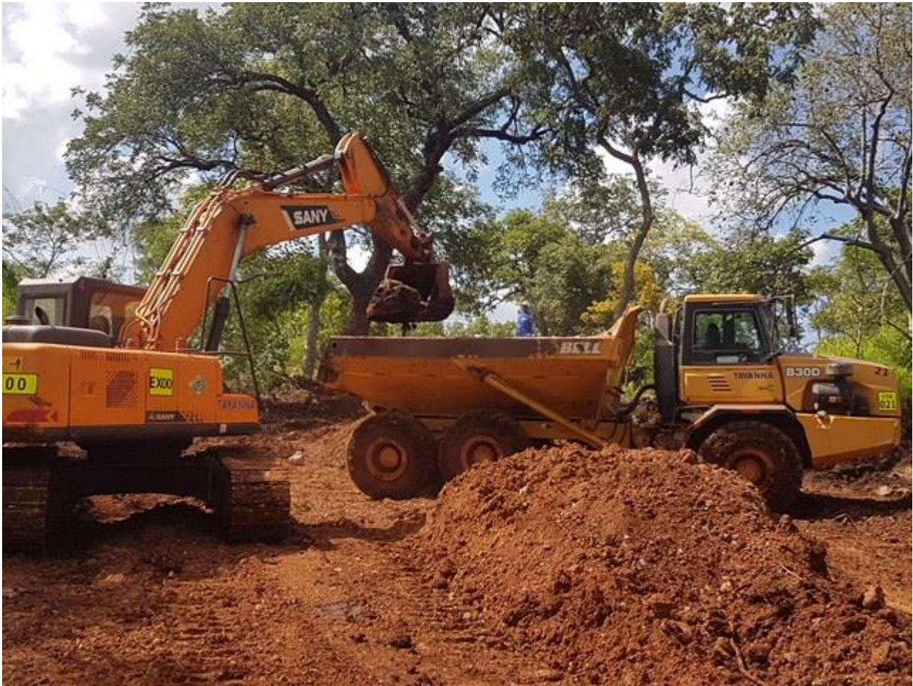
Montepuez Graphite Project: siteworks
