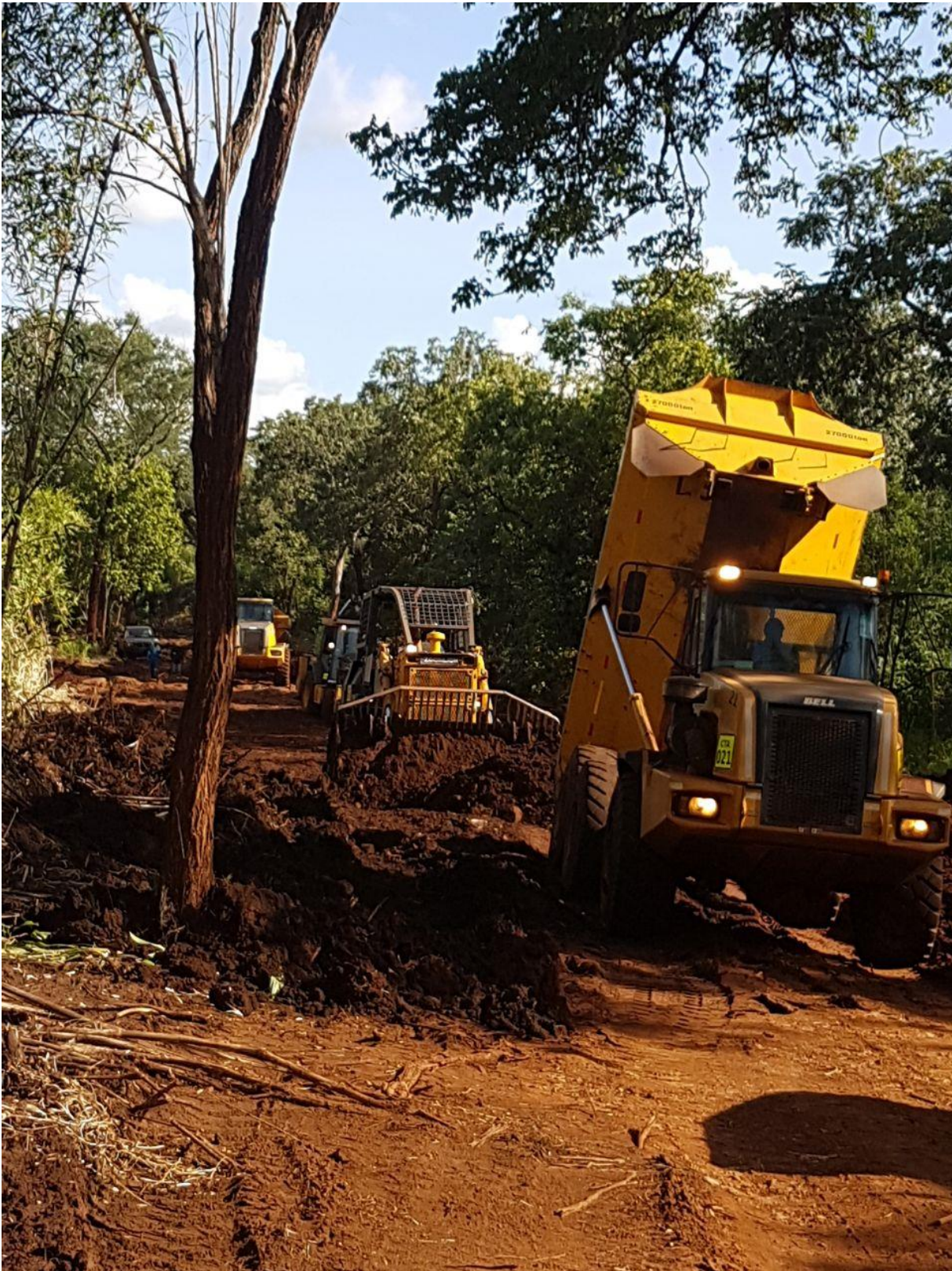
Montepuez Graphite Project: Roadworks
